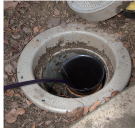
Insert Sleeve in cleanout
